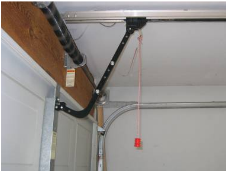
Electronic Garage Door Release (In the manual position)
